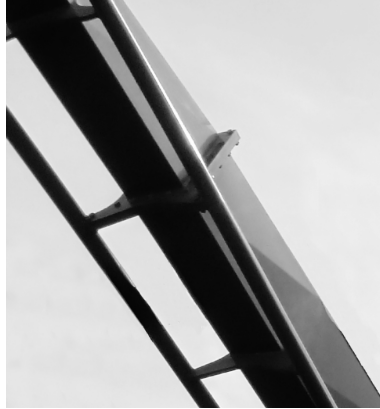
Figure 5.8: A detail of track profile of Nemesis - an inverted roller coaster in Thorpe park, UK.
