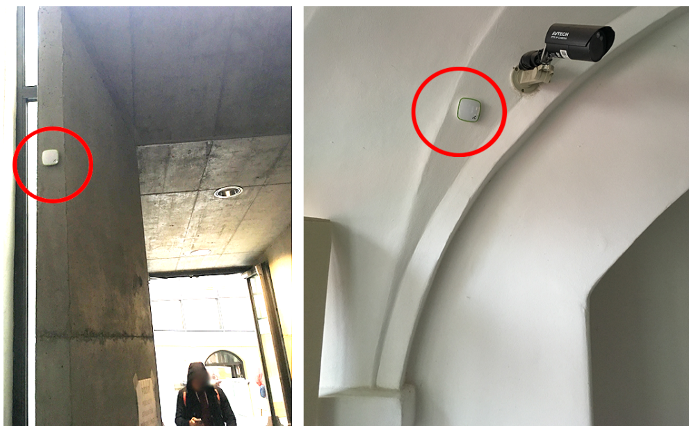
Figure 7 Beacons installation at the suitable places.
